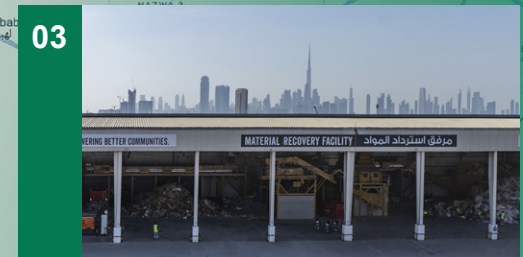
MATERIAL RECOVERY FACILITY (MRF)
