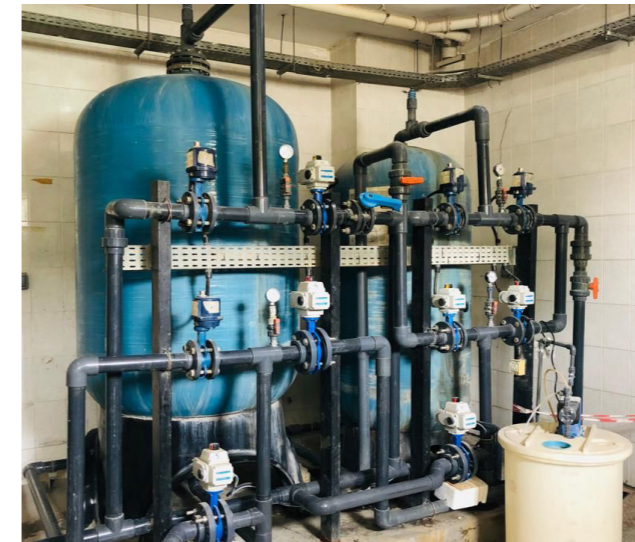
Grey Water Recycling at DulSCO Village Accommodation
